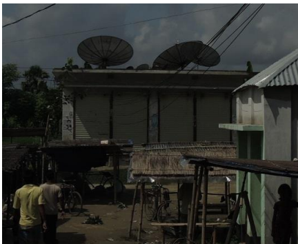
The dish-line is a cable TV company that captures channels with satellite dishes ...
